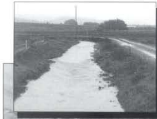
Figure 1. Typical trapezoidal channel in photo (left) became a larger and often less efficient channel (below) to meet environmental concerns.
