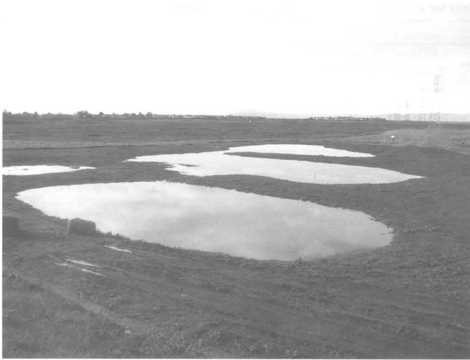
Figure 3. A typical seasonal marsh restoration project, just after final grading.
