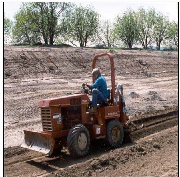
Construction of mitigation wetlands at Laguna Creek, Sacramento.
